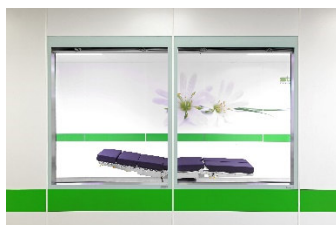
Design example: Flush window. Fully open - blind partially open - blind closed (from left to right)
